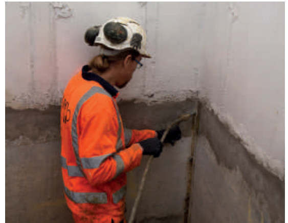
PU waterproofing injection in a lift shaft
