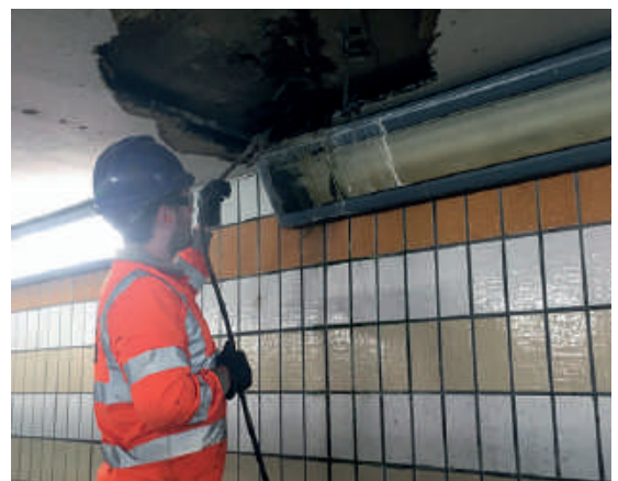
Waterproofing injection in an underpass
