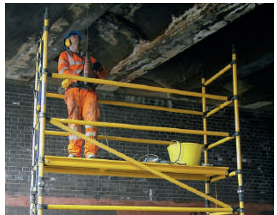
Acrylic waterproofing injection to a bridge soffit
