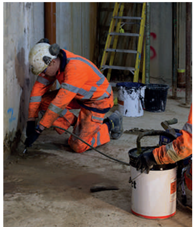
Leaksealing injection between floor slab and wall
