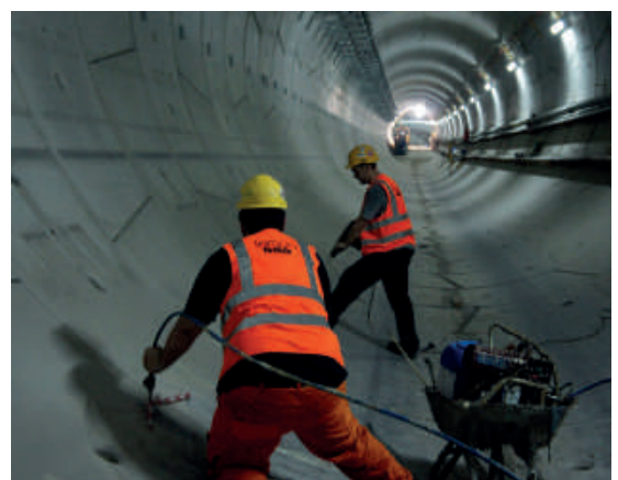
PU gasket injection in a segment tunnel
