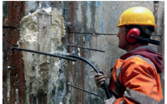
PU injection to consolidate before header opening
