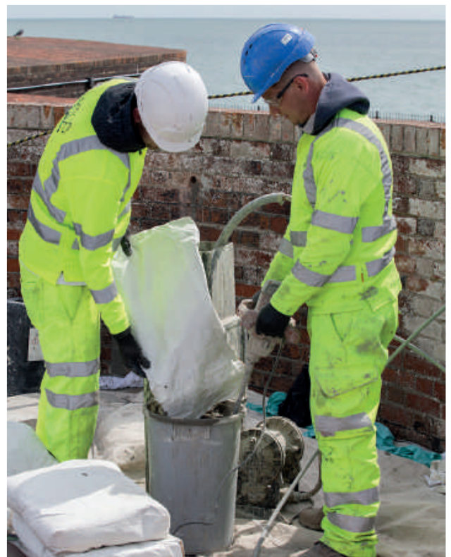
Loading the pump hopper with lime grout
