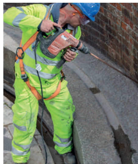
Lime injection through the parapet
