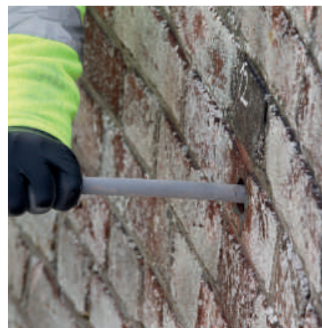
Feeding in the injection hose
