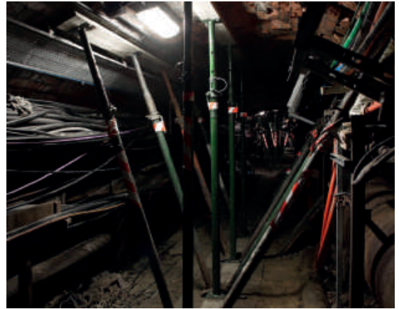
Temporary works: radial propping to damaged brick tunnel
