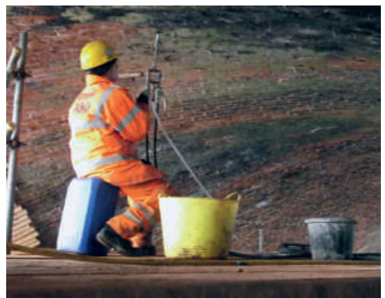
PU strengthening injection to a flood defence structure
