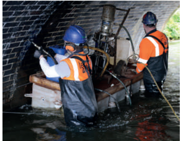
Acrylic waterproofing injection off a raft
