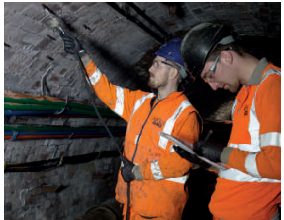
PU waterproofing injection and noting of quantities
