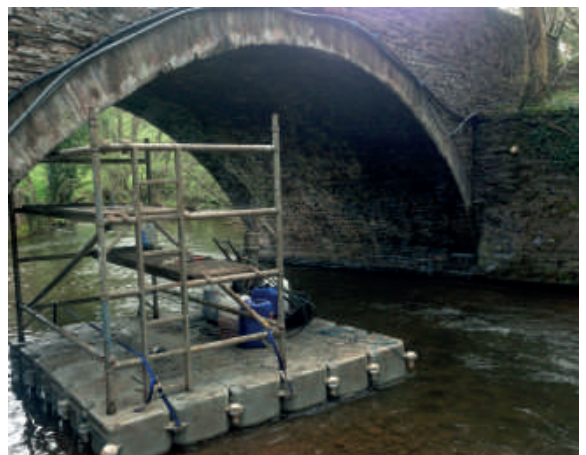
Raft being set up for waterproofing injection over a watercourse
