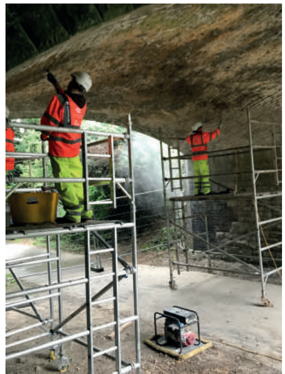
Pointing before waterproofing injection
